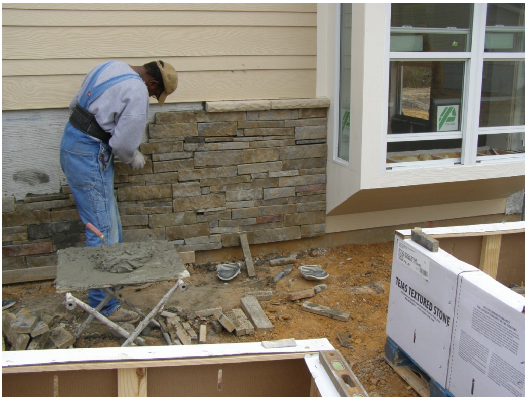
Manufactured stone going up
