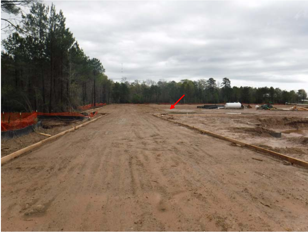
9. Viewing the stabilization and perimeter forms installed at the north drive.
