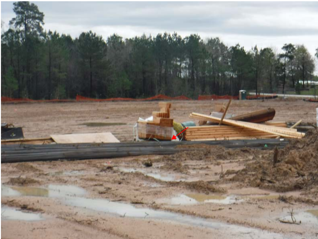
10. The reinforcing steel and forming materials stored onsite.
