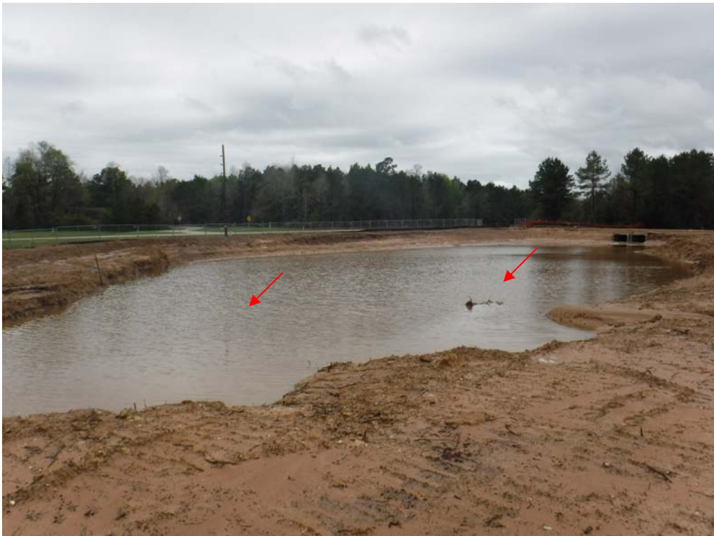
6. Excavation of the detention pond is in progress.
