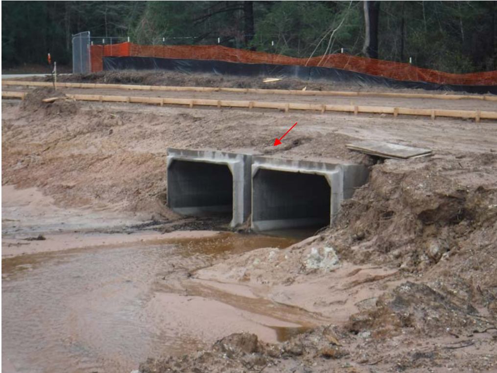
7. Installation of the two large drainage boxes is complete at the detention pond.
