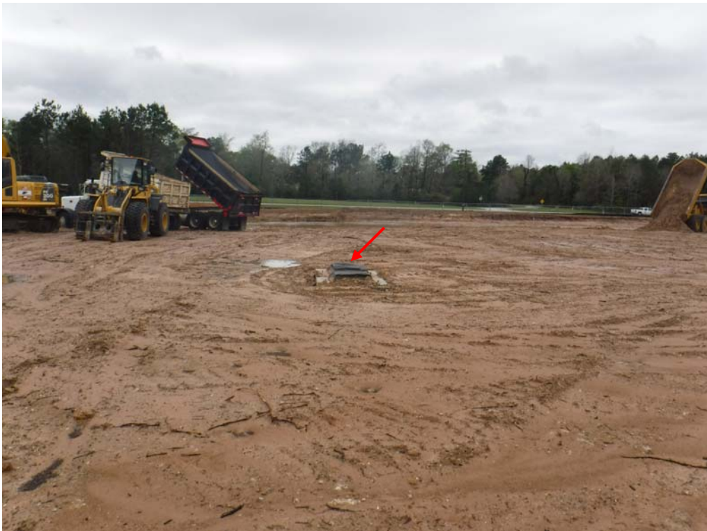
8. Installation of the inlet boxes and storm drainage piping is in progress at the paved areas.
