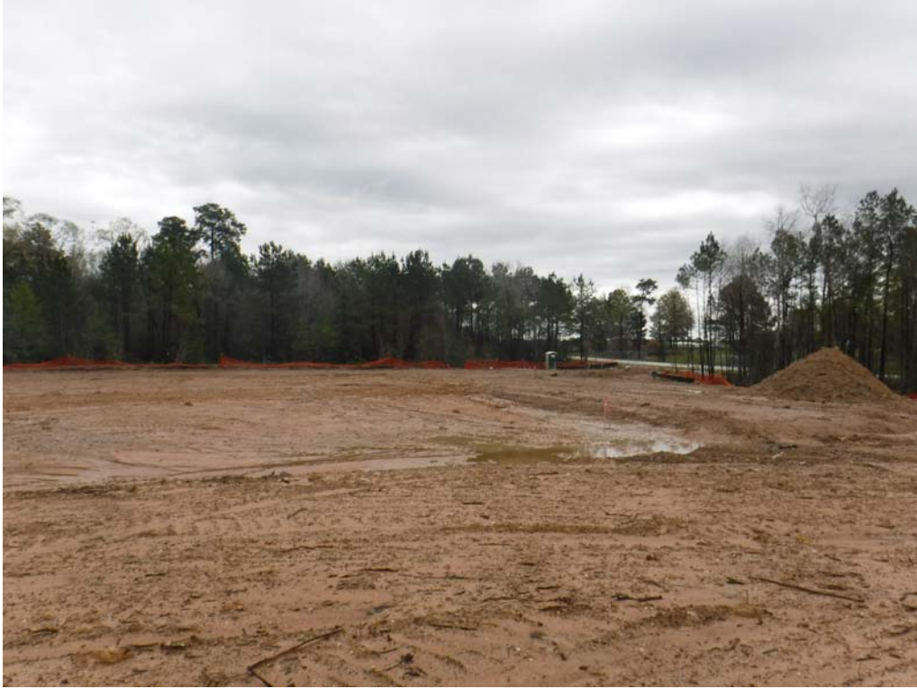
5. Clearing and grading has been completed with work on the building pad underway.
