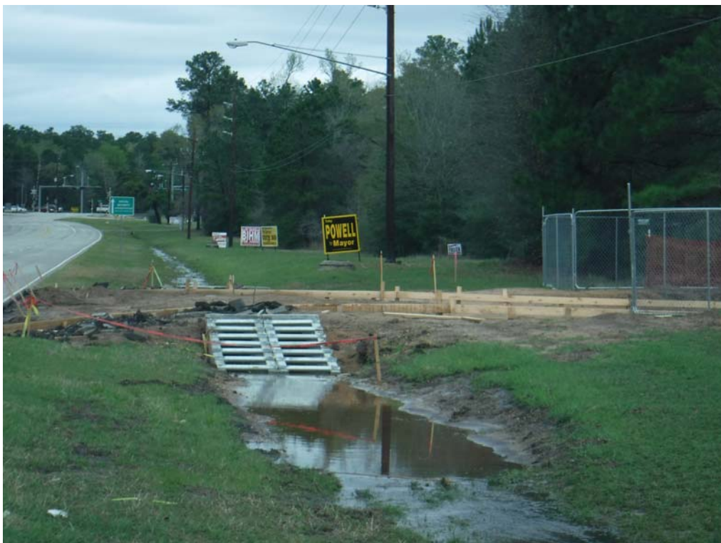
2. Viewing the culvert pipe and safety end installed at the entrance off St. Ed Holcomb Boulevard.
