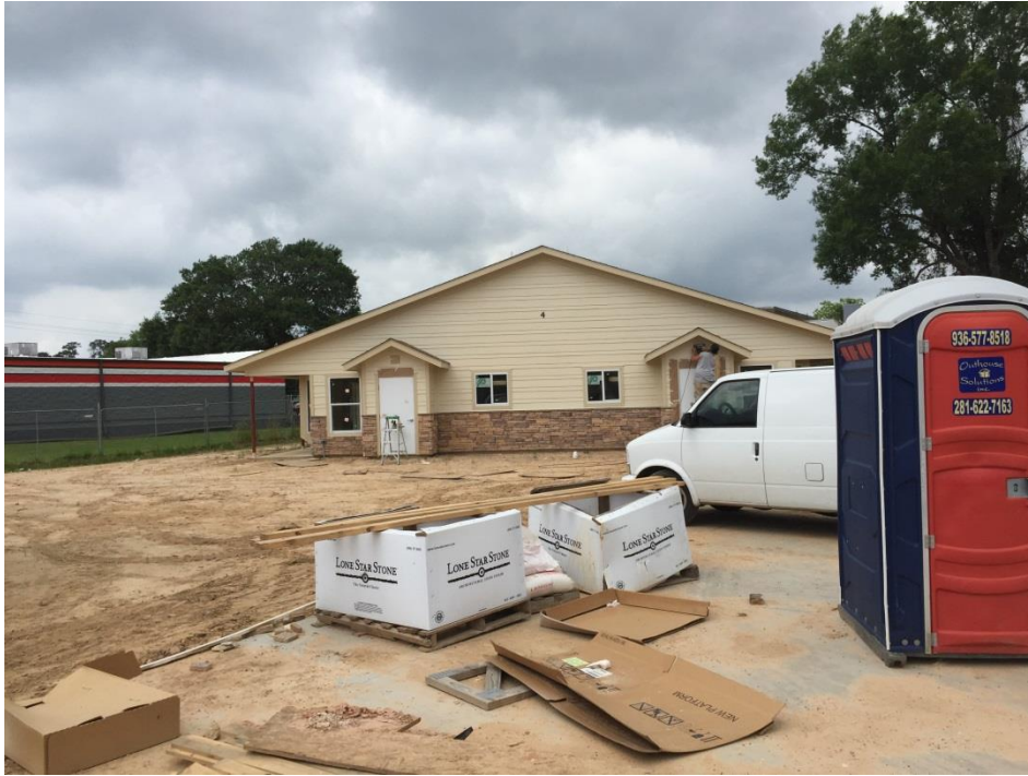
Exterior of Building 4
