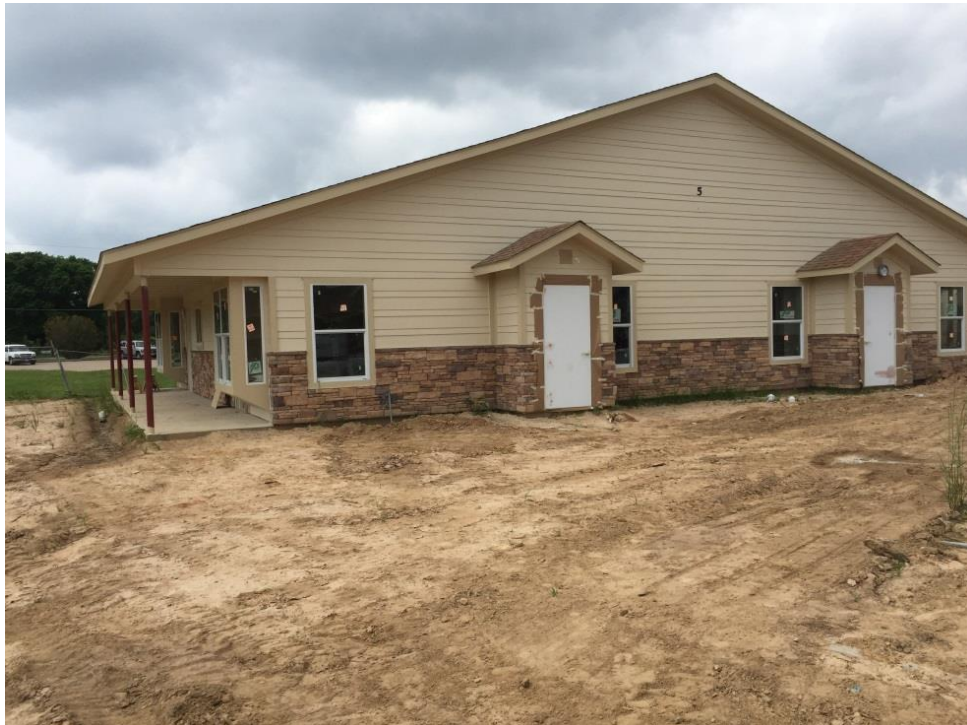
Exterior of Building 5
