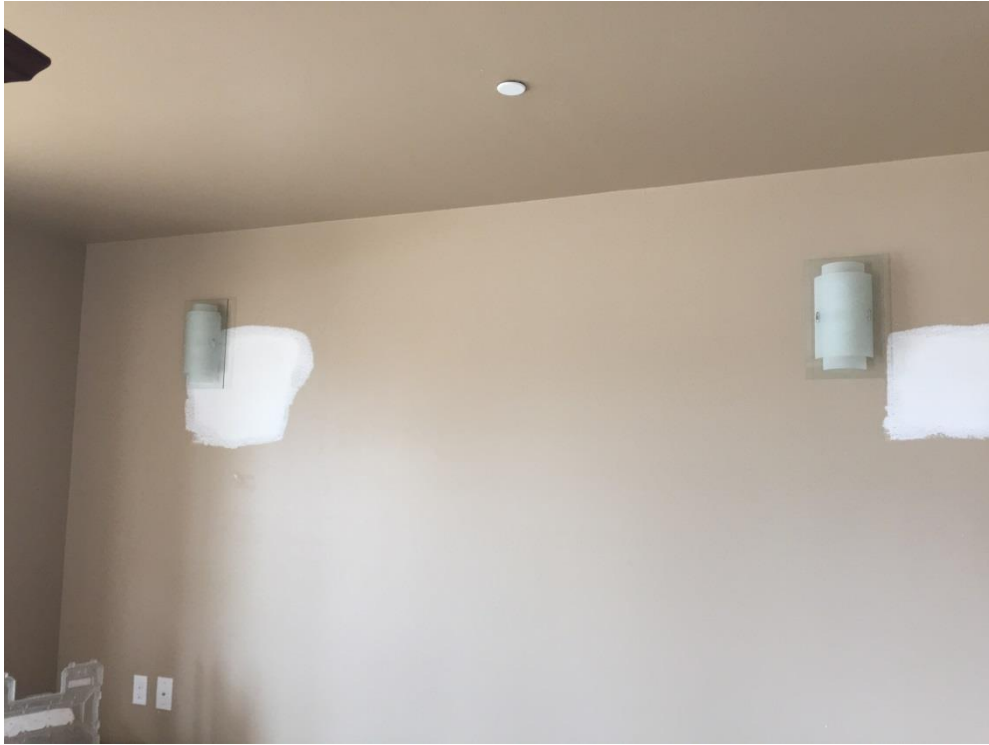
Interior Building 2- Wall Sconces
